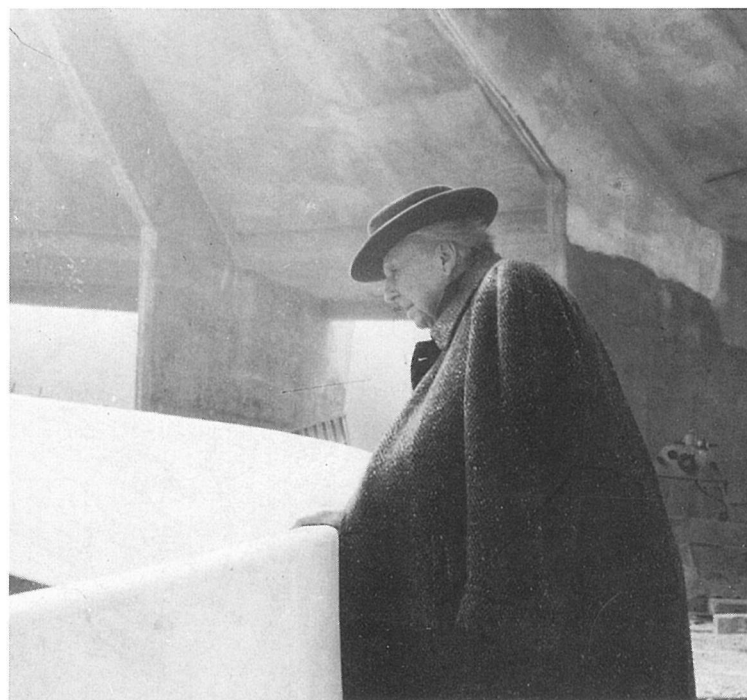
11. Frank Lloyd Wright on the museum's top ramp during construction.
